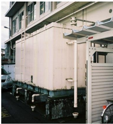
Picture 11 General government office (Tokamachi City) Point E in the figure: Intensity 6, upper division
