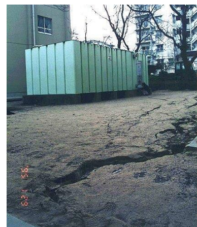
Picture 9 Municipal junior high school (Higashi-Nada Ward, Kobe City) Point C in the figure: Intensity 7
