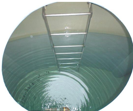
Picture 18 Picture of inside of water tank taken from a manhole
